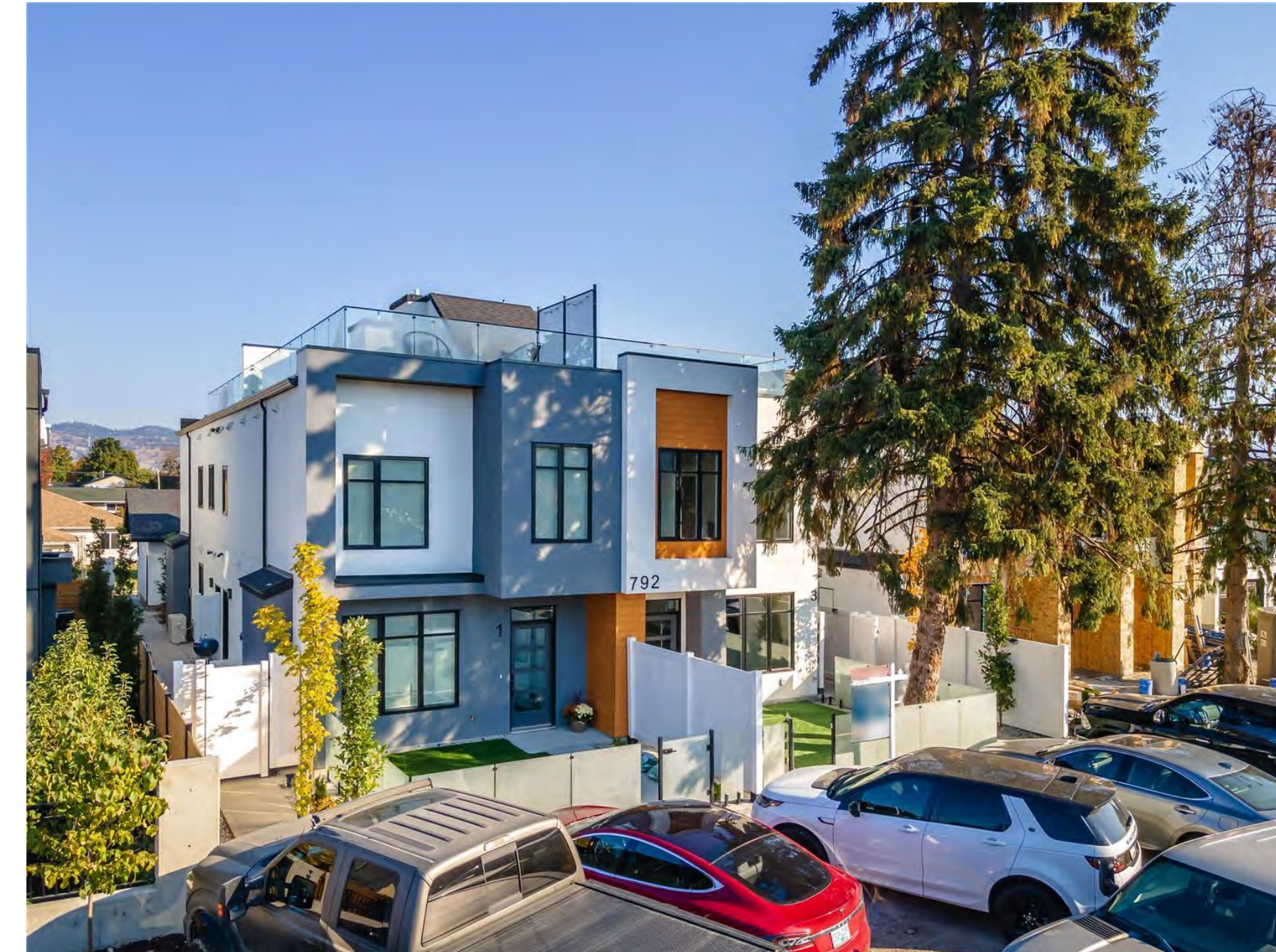
PRECEDENT IMAGE: 1.8M HT WHITE VINYL FENCE W/ 1.2M HT GLASS RAILING.
